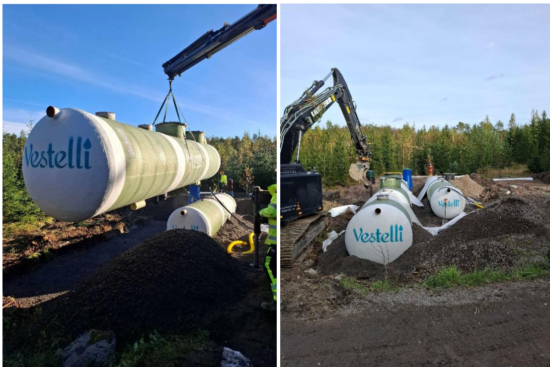
Picture 4. The process tank was lifted into position, anchored and connected to the previously installed infrastructure.
