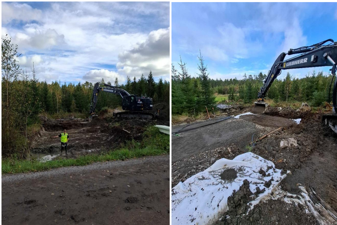
Picture 3. Preparatory earthworks undertaken by Maanrakennus Marela Oy
