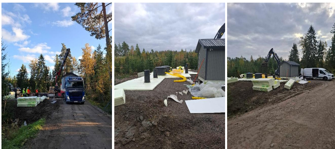
Picture 5. Installation of the service building.
