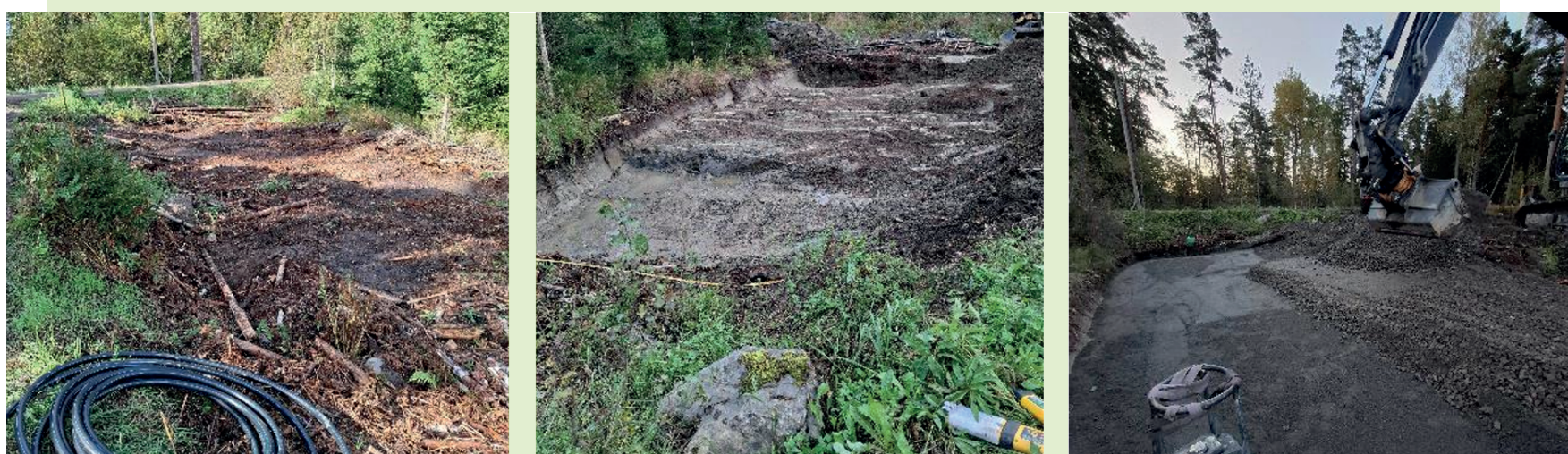
Preparation of the sedimentation and process tank sites, 22 September 2025
