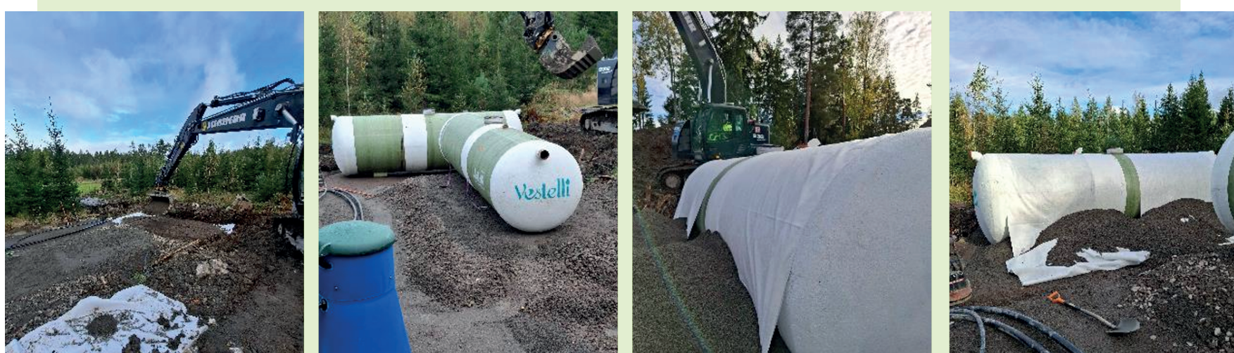
Placement of the overflow and sedimentation tanks, 23 September 2025
