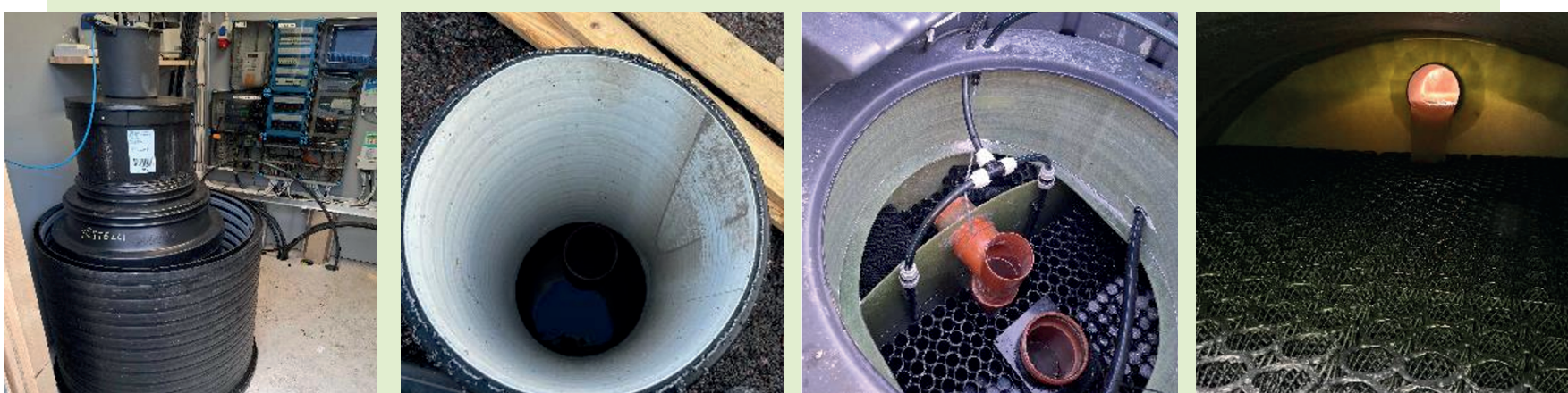
Start-up of the biological treatment process, 6 October 2025
