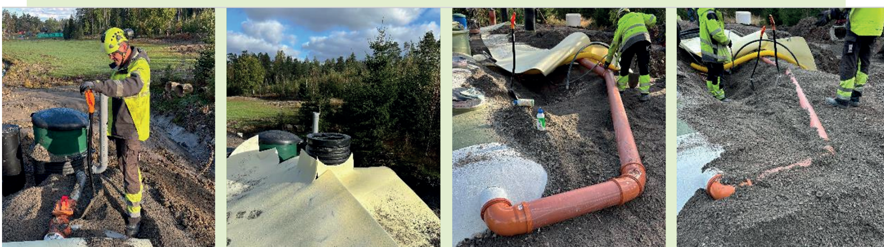
Completion of tank connections, 30 September 2025
