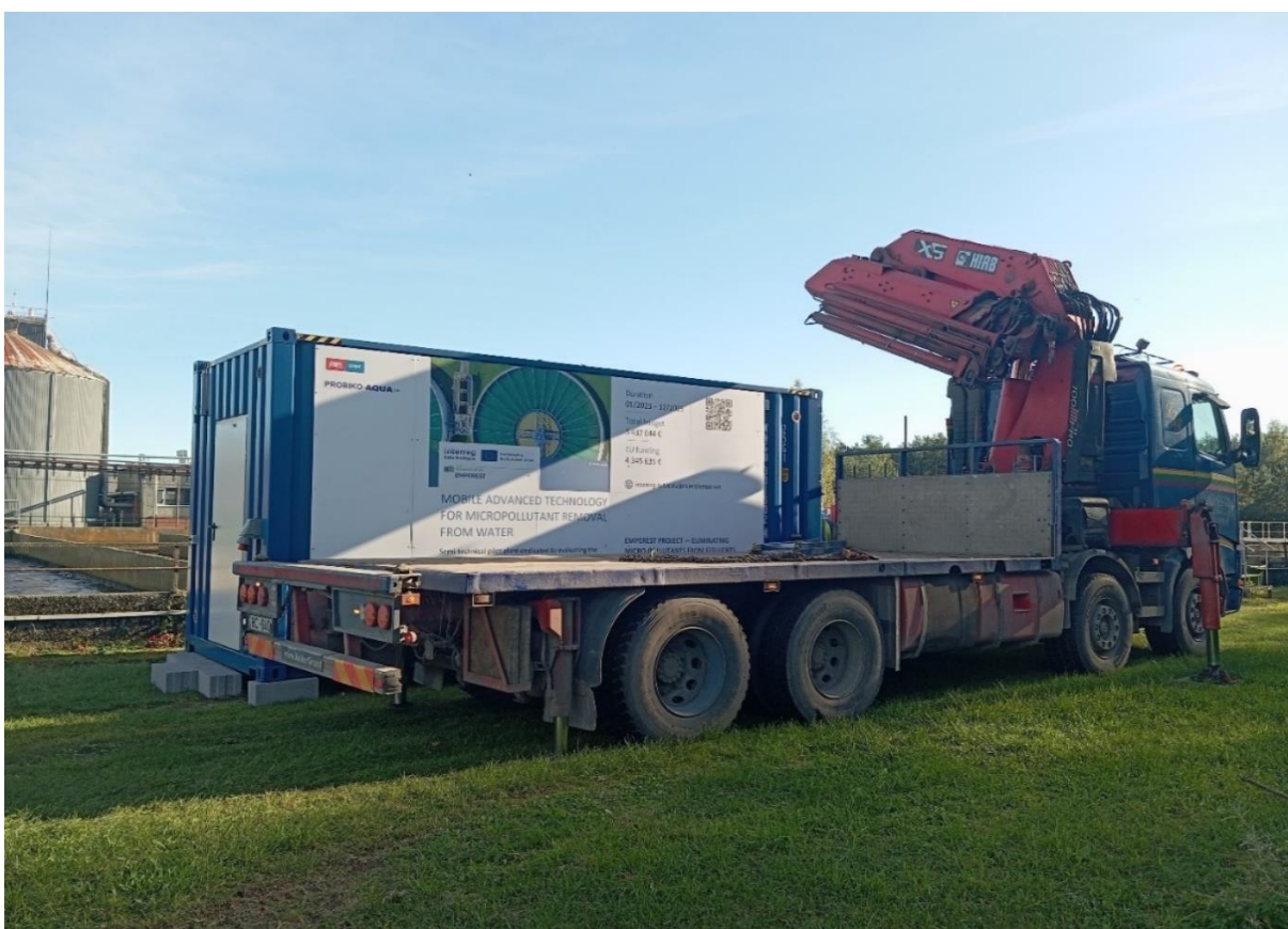
Fig. 1 View of the pilot plant located at the Daugavgrīva WWTP.
