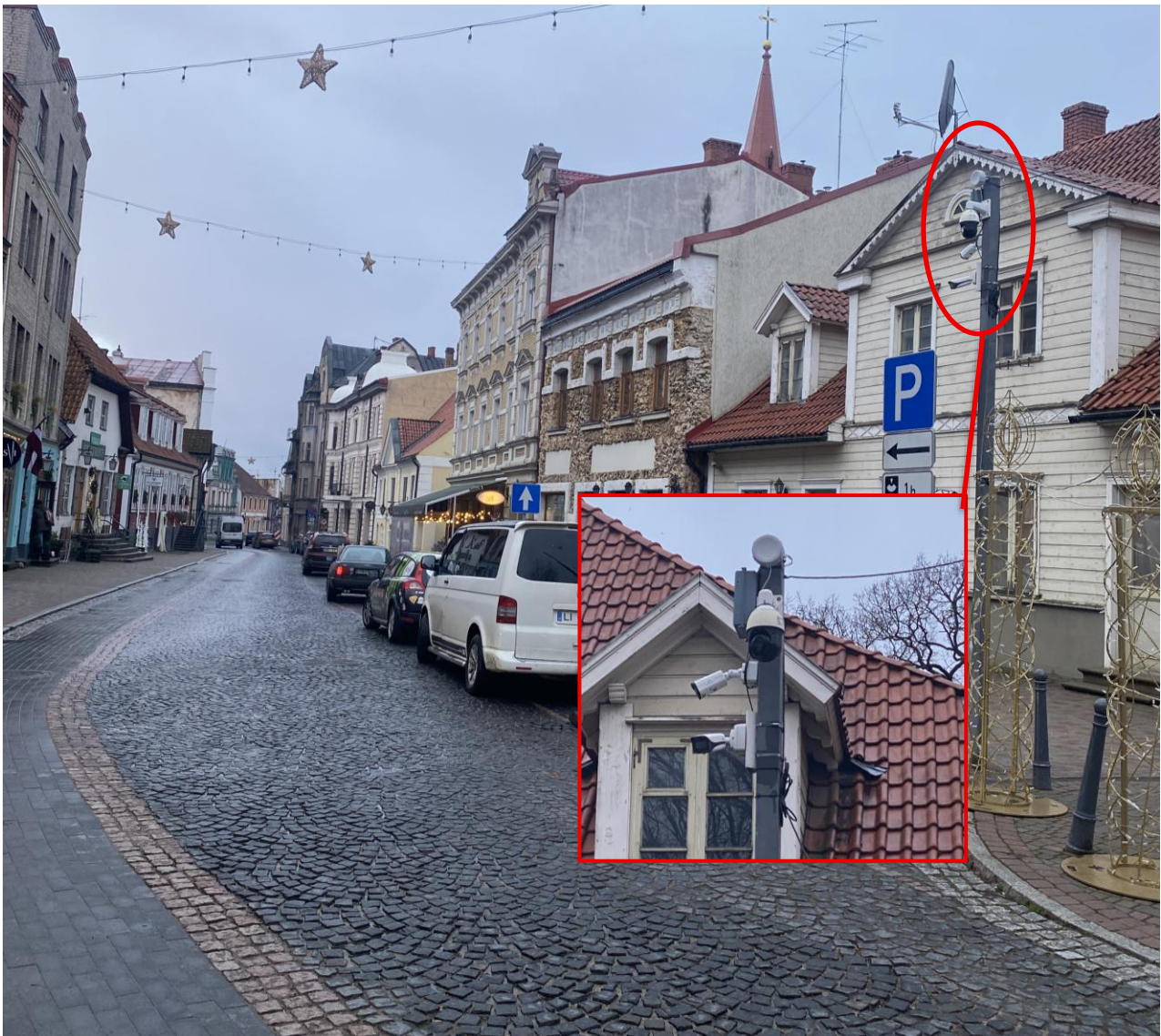
Figure 3. AI supported camera. Source: Cēsis Municipality.
