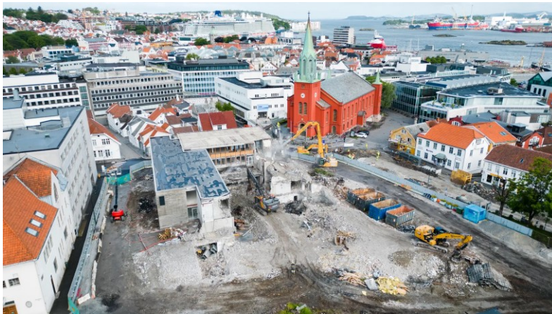
Figure 7. Nytorget – Start of demolitions (source: Stavanger Aftenblad)
