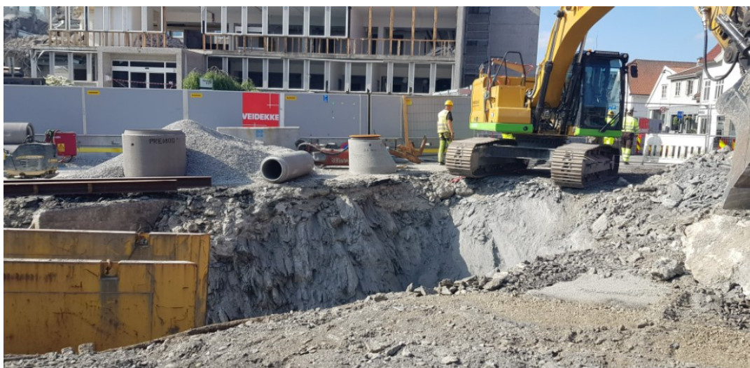
Figure 8. Nytorget – Old pipelines replacement (source: Stavanger Kommune)
