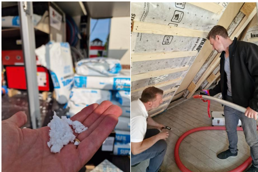
Figure 3: Blown In insulation installation © ZEBAU GmbH
