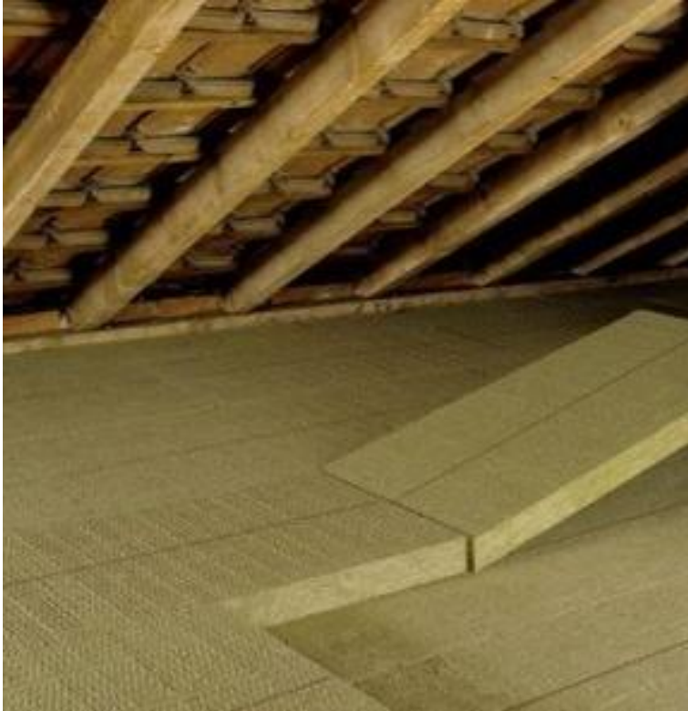
Figure 1: Insulation example on top floor © ZEBAU GmbH
