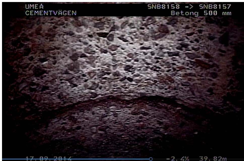
Figure 23. Degradation of concrete pipe due to \text{H}_2\text{SO}_4 formation from \text{H}_2\text{S} .
