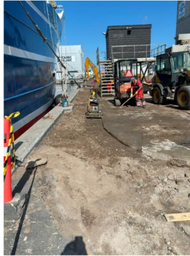
Construction work - cable trenching and routing.
