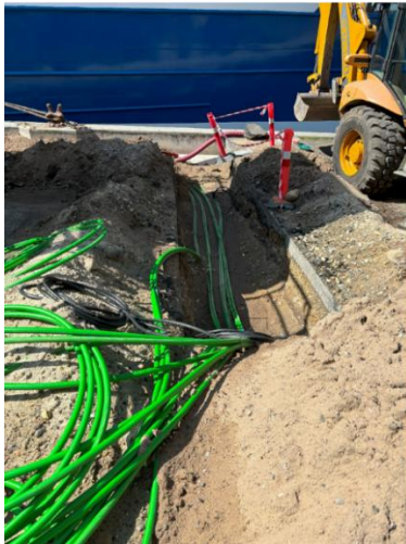
Construction work - cable trenching and routing.
