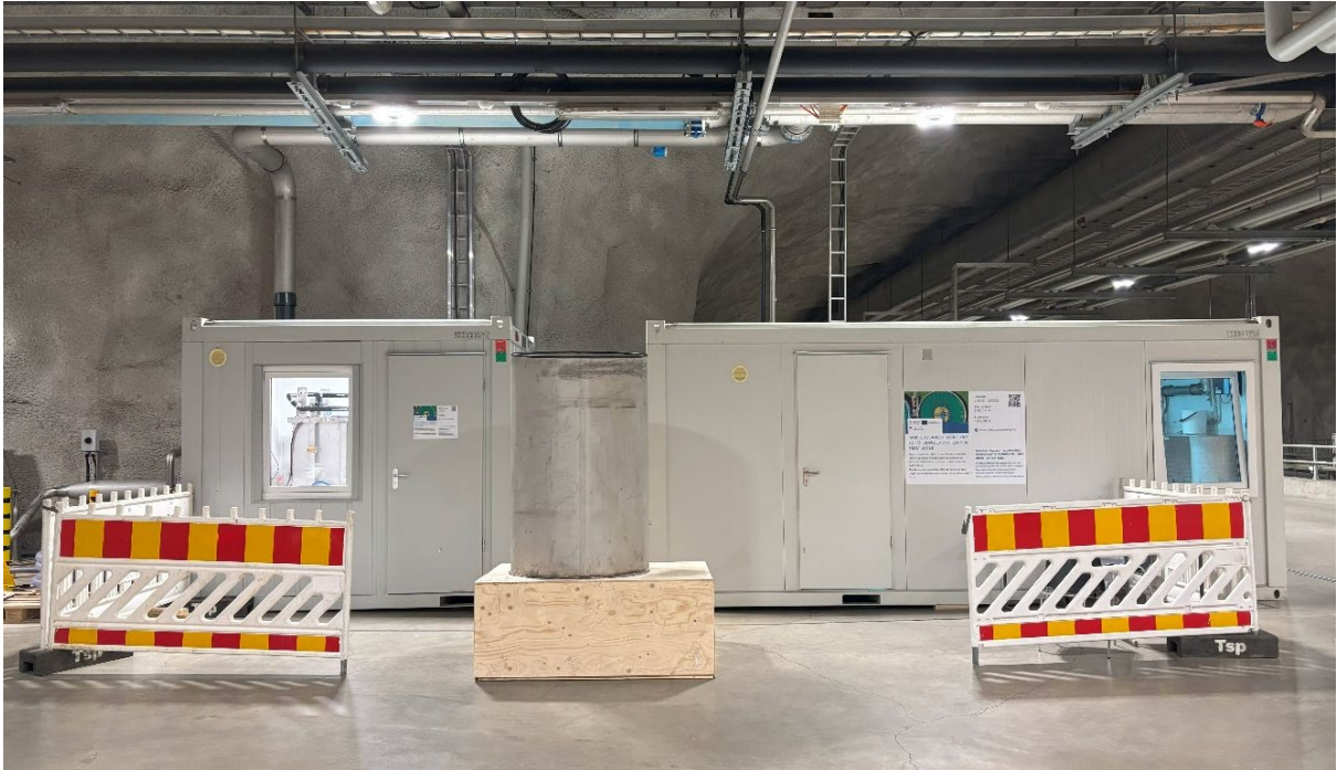
Figure 1: View of the pilot plant located at the Turku region WWTP
