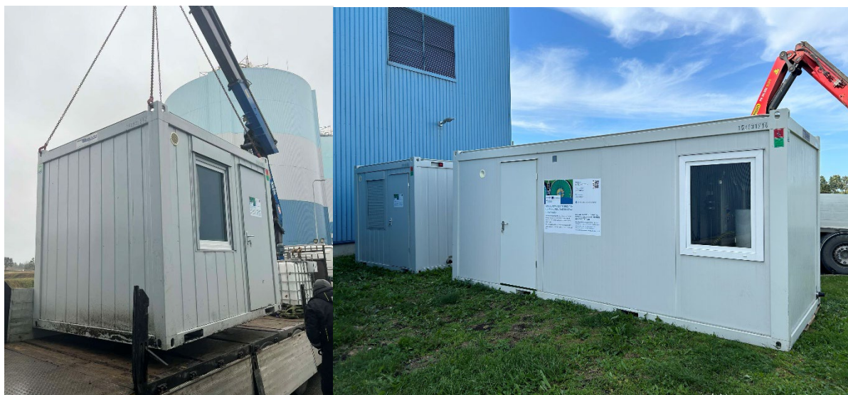
Figure 2. View of the pilot plant (two sea containers) located at the Tallinn WWTP in Estonia
