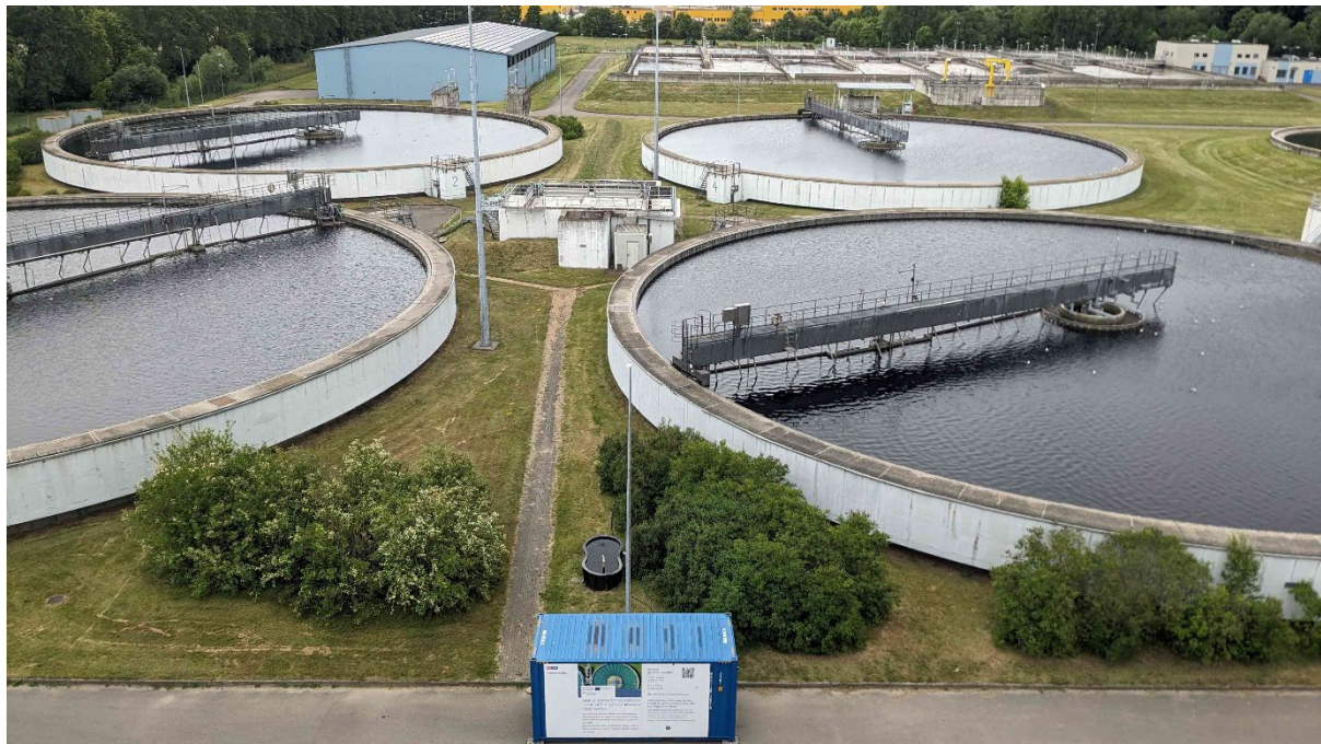
Figure 2. View of the pilot plant located at the Kaunas WWTP.
