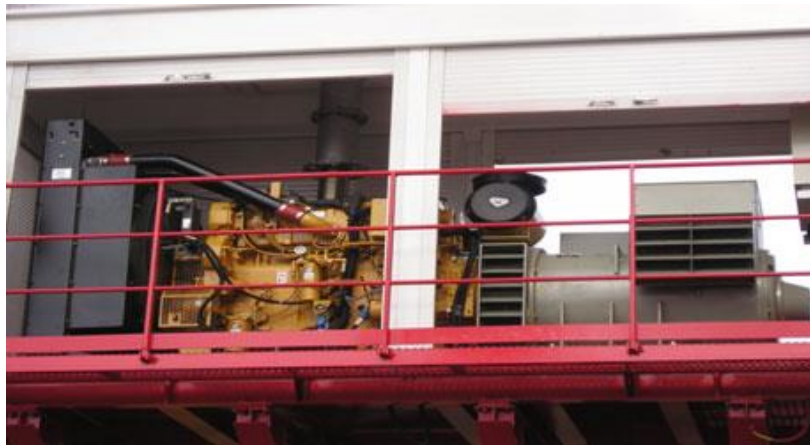
Fig. 10. Diesel generator set [Handbook of Port Machinery, 2024]
