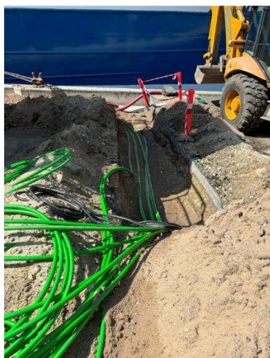
Construction work - cable trenching and routing.
