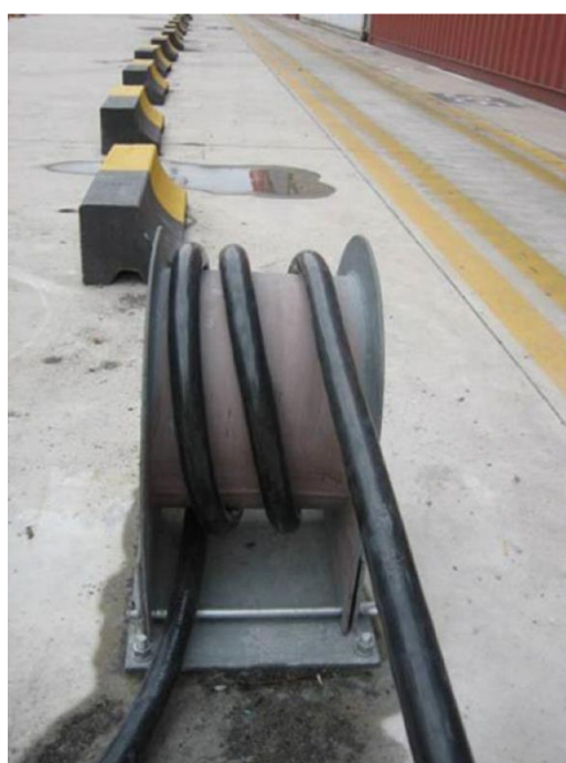
Fig. 14. Power supply cable ground fixing device [Handbook of Port Machinery, 2024]
