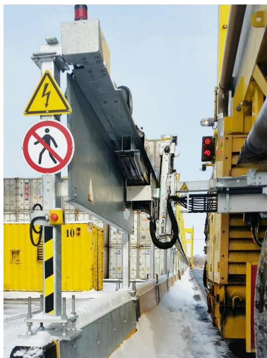
Fig. 16. Example of Conductor Bar RTG supply system [Conductix wampfler information materials]
