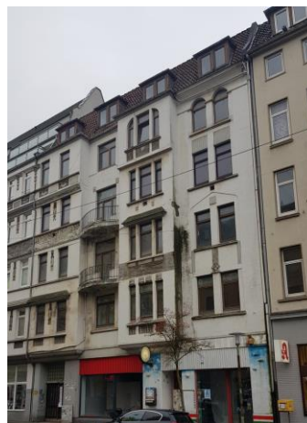
Picture 2: unrenovated buildings ©KEEA
