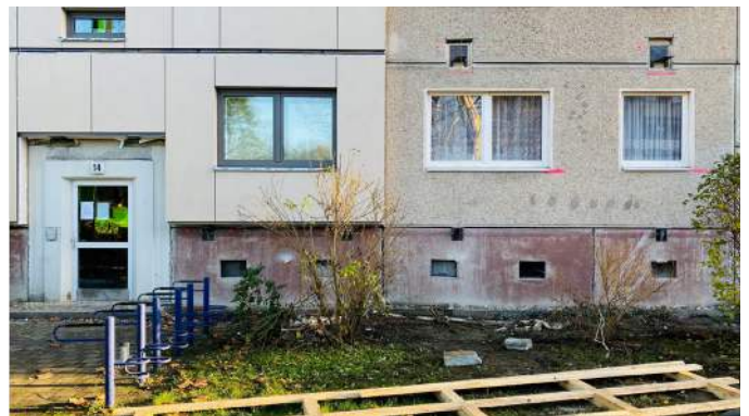
Figure 8: Before and after an installation of a prefabricated element. Source: Seeria Renova
