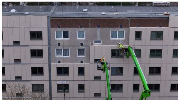
Figure 7: Construction works at the panel building in Ludwigsfelde, Copyrights: Seeria Renova
