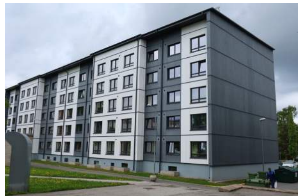
Figure 3. The pilot building before and after renovation. Source: K. Kuusk, P. Pihelo, and T. Kalamees, “Renovation of apartment buildings with prefabricated modular panels”, in: E3S Web of Conferences, vol. 111, p. 03023, January 2019, doi: 10.1051/e3sconf/201911103023.
