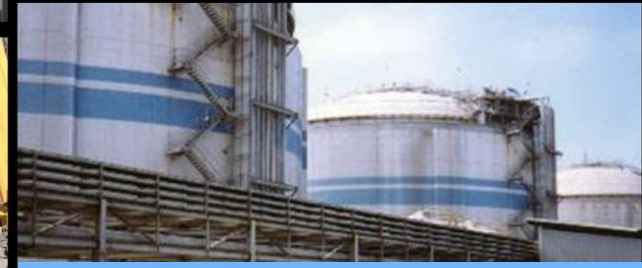
Formosa Petrochemical Corporation, Mailiao, Taiwan Ammonia Terminal incl. 2 x 30,000 m 3 Tanks
