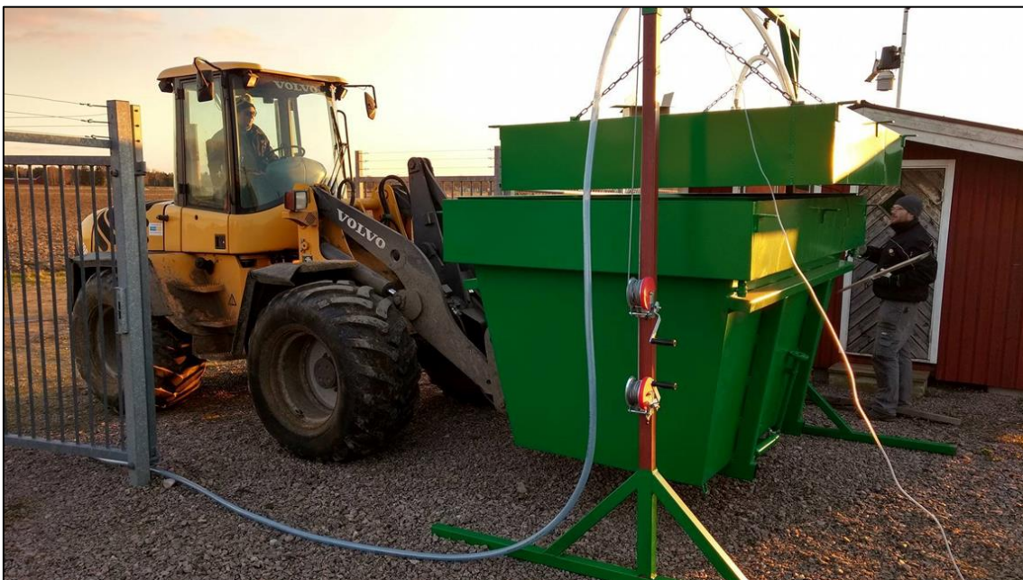
Figure 11: Positioning of ash filter container at pilot plant Sötåsen (RISE)
