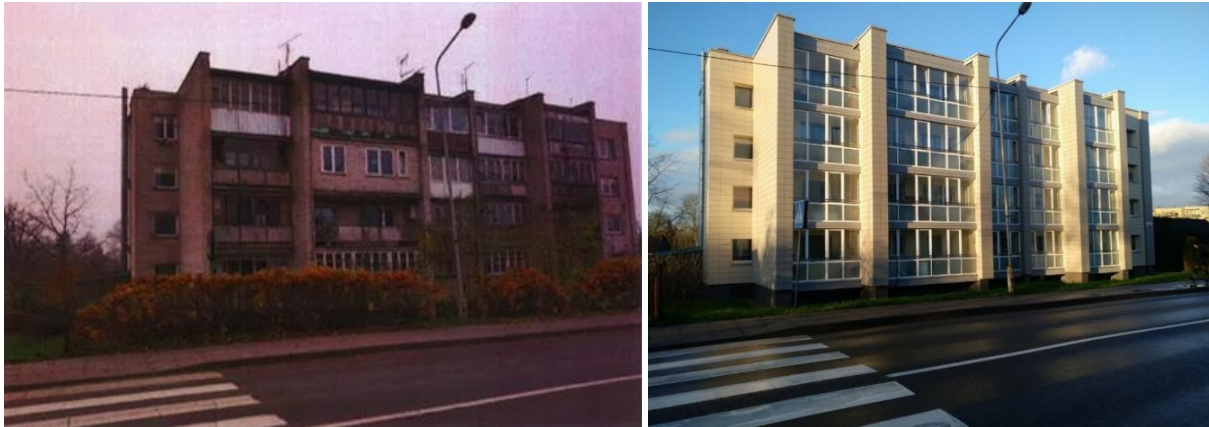
Figure 2. Before modernization (a)
