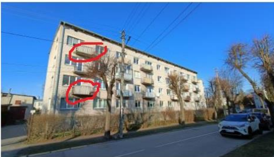
Fig. 5. Balcony PV in Kaunas
