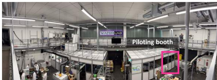
Pictures 1. Savonia UAS. WaterLAB. ReNutriWater Project. Piloting 2024. Disinfection station.
