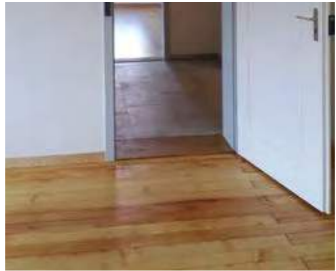
Figure 4: Historic fir plank floor sanded and oiled (Photo Auraplan),
