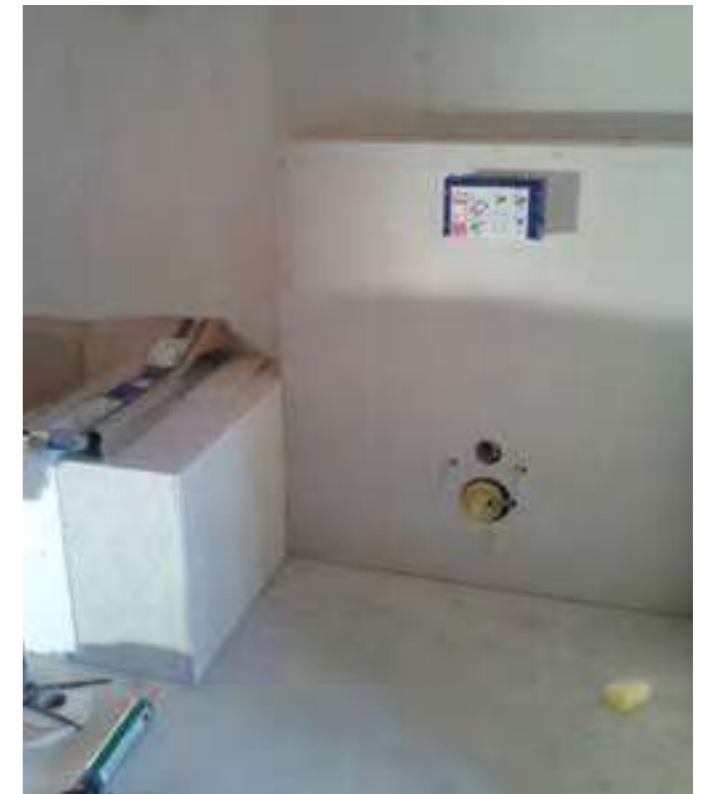
Figure 7: Fermacell planking in the bathroom (Photo Auraplan)
