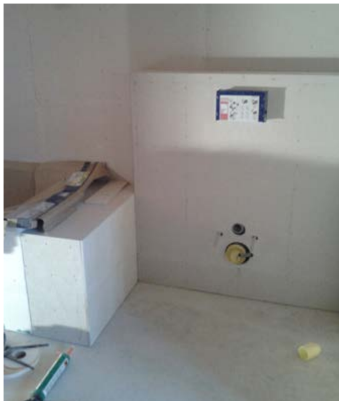
Figure 7: Fermacell planking in the bathroom (Photo Auraplan)
