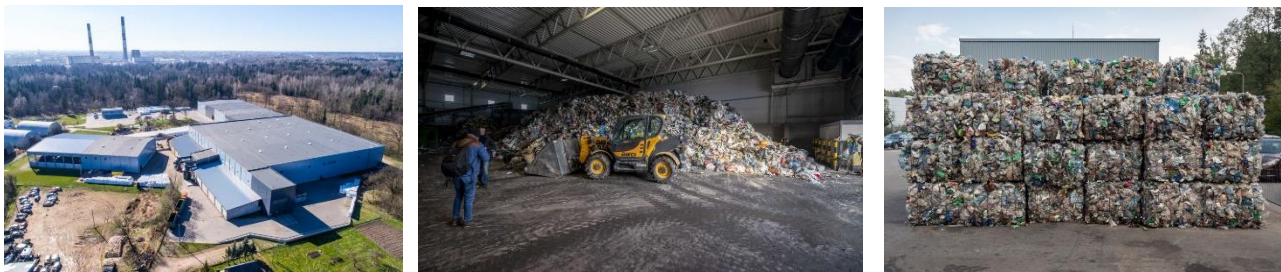
Fig.7 Kaunas MBT facility
