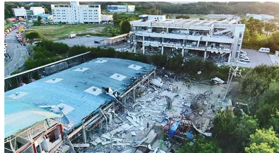
Station explosion in Norway 10.06. 2019 The cause - a hydrogen leak from the high-pressure store - was caused by an incorrectly fitted connector.
