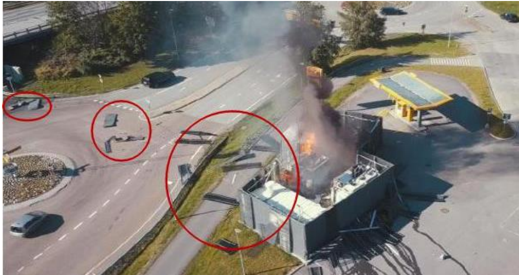
Explosion of P2G hydrogen test plant in South Korea 23.05.2019 Cause - oxygen has entered the hydrogen tank
