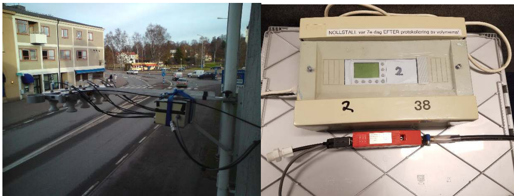
Sampling heads on a façade.
