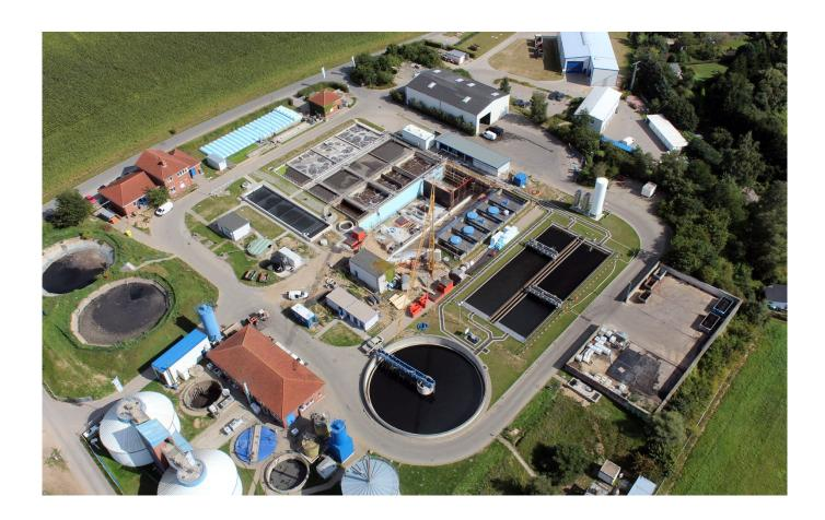
Optimization potentials are identified based on a successful calibration and validation of the simulation model including pre-treatment, aerobic biological treatment, sludge digestion, co-fermentation, thermal hydrolysis and deammonification. Subsequently, the findings are implemented in the full-scale operation of the treatment plant. The verification process includes a detailed measurement campaign before and after implementation of the optimization actions.
