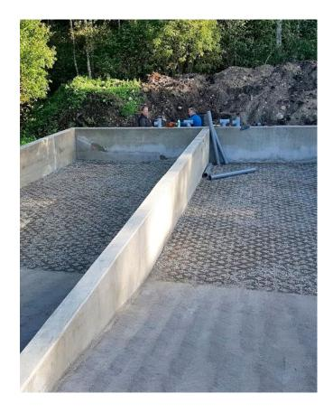
on preceding studies is an essential part of the piloting process. The humification beds in Türi and Oisu were constructed next to the wastewater treatment plants and they have the same working principle, while their structure is a bit different in order to determine the most feasible practice.
